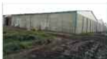
7,000m 2 closed + 33,000m 2 open warehouse at port of Douala area (Kinshasa)
